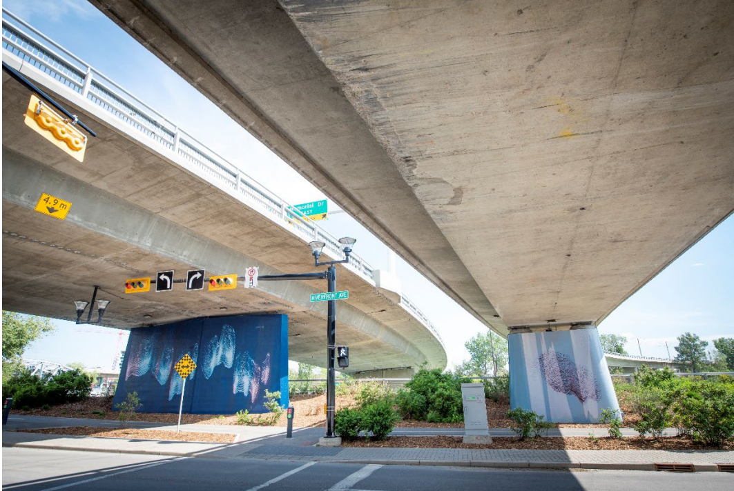
Abutment B + C, facing south
